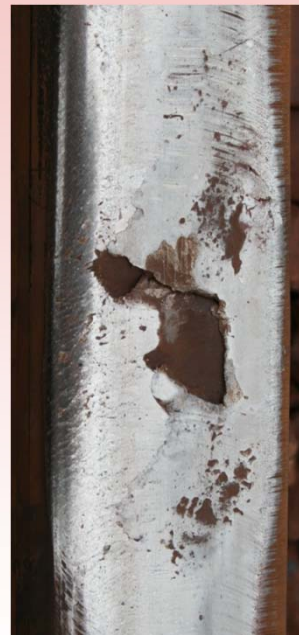
Fully Grown Cracks
